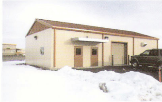
Hazardous Material Storage
